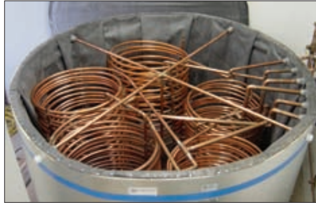
An above-tank view shows the innards of the storage tank complete with coils.
