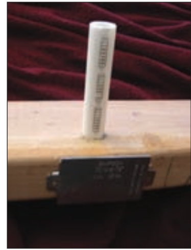
A nail stop prevents a trim nail from penetrating a PEX tube passing through a stud.
