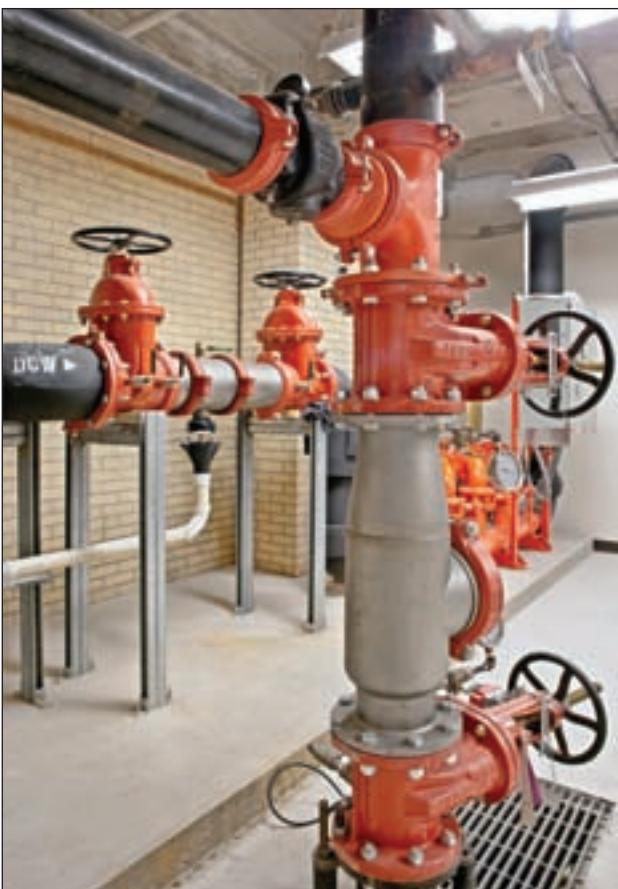
*Four and eight-inch Watts model 957 RPZ backflow preventers protect the domestic water system. Strainers installed upstream of the RPZs help keep debris from getting into the OneFlow system and backflow preventers.*
