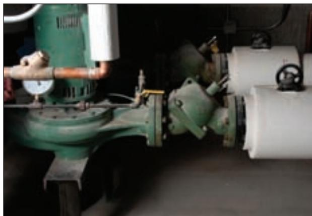
*This Taco vertical in-line pump resides on Aqua's 57th floor. It circulates hot water for fan coil units to condo fan coil units at that level, and to living spaces in the floors above it.*
