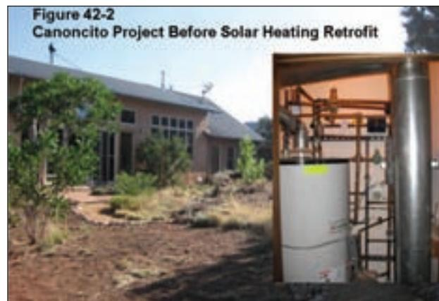
The only heating fuel available is propane, and the original gas burner was a Lochinvar DDL075 that provided both potable DHW and boiler fluid for the floors (seen on the right in Fig.42-2). This resembles a conventional 75-gallon gas water heater tank, but has a heat exchanger coil built into it, so that boiler fluid
